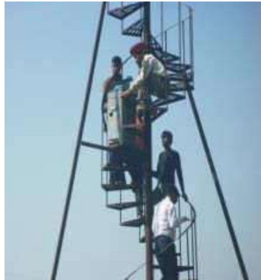
Fig.6.14 Near ETP Plant
