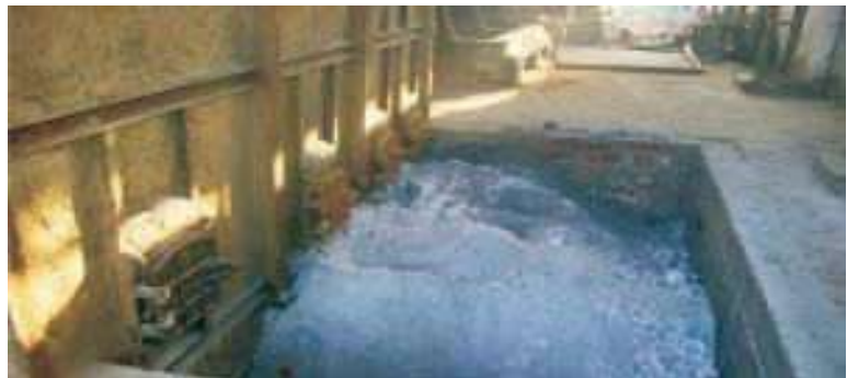
Fig 4.15-Partially covered storage of husk fired boiler ash
