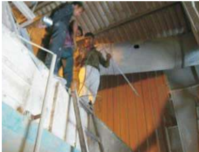
Fig.6.4 Port Hole at Cyclone inlet
