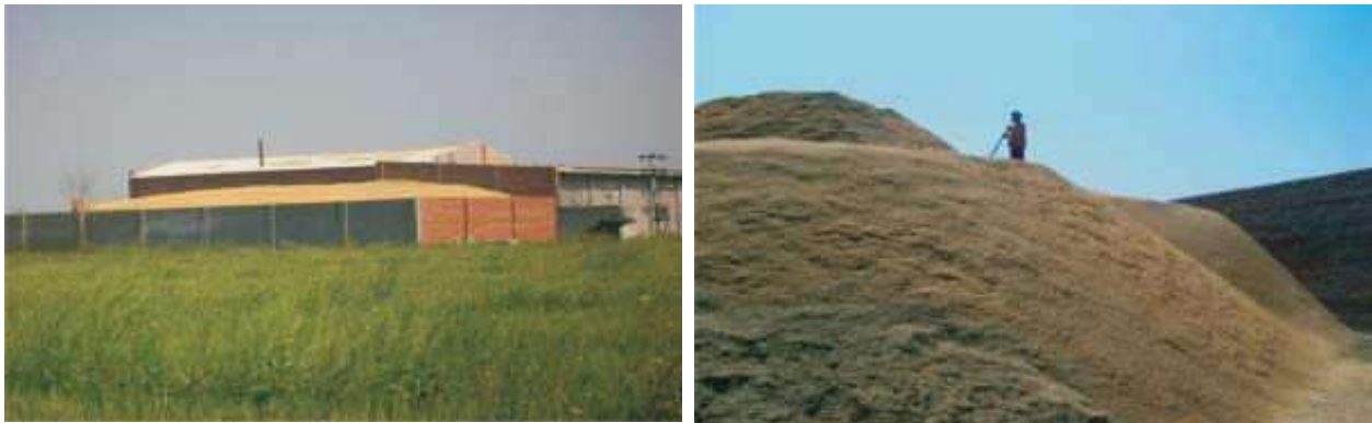
Fig 4.6-Rice husk storage in fully open area with boundary walls
